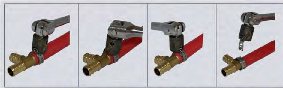
Slide tool over clamp ear
